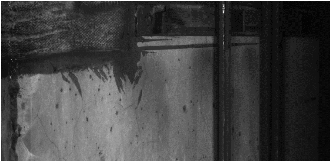
Fig. 3. Original image of the tunnel
