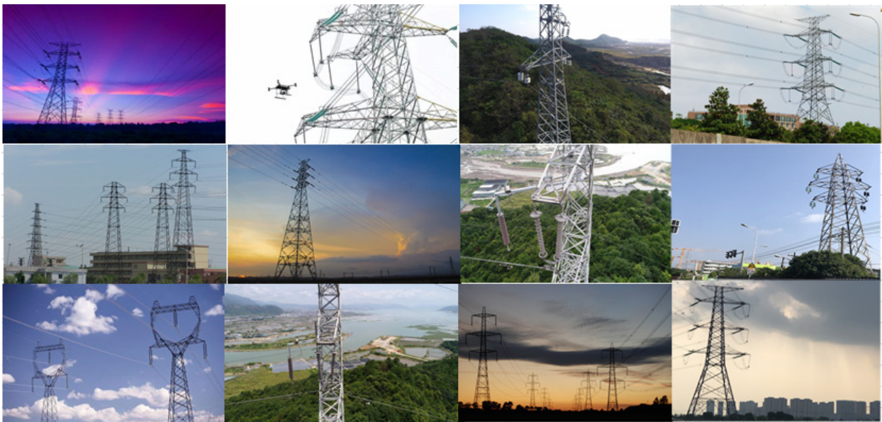
Fig. 2. Partial transmission towers and insulators
